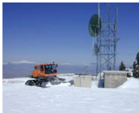
Snowcat at the 146.66 repeater on skyline
